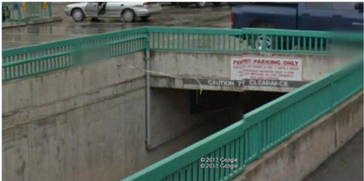
Photo 21: Parking Garage Close up
