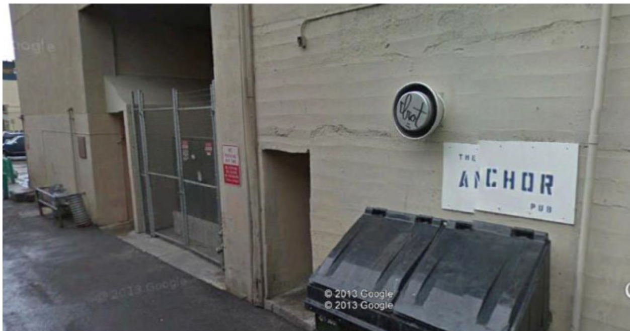
Photo 29: South Wall of Anchor Pub
