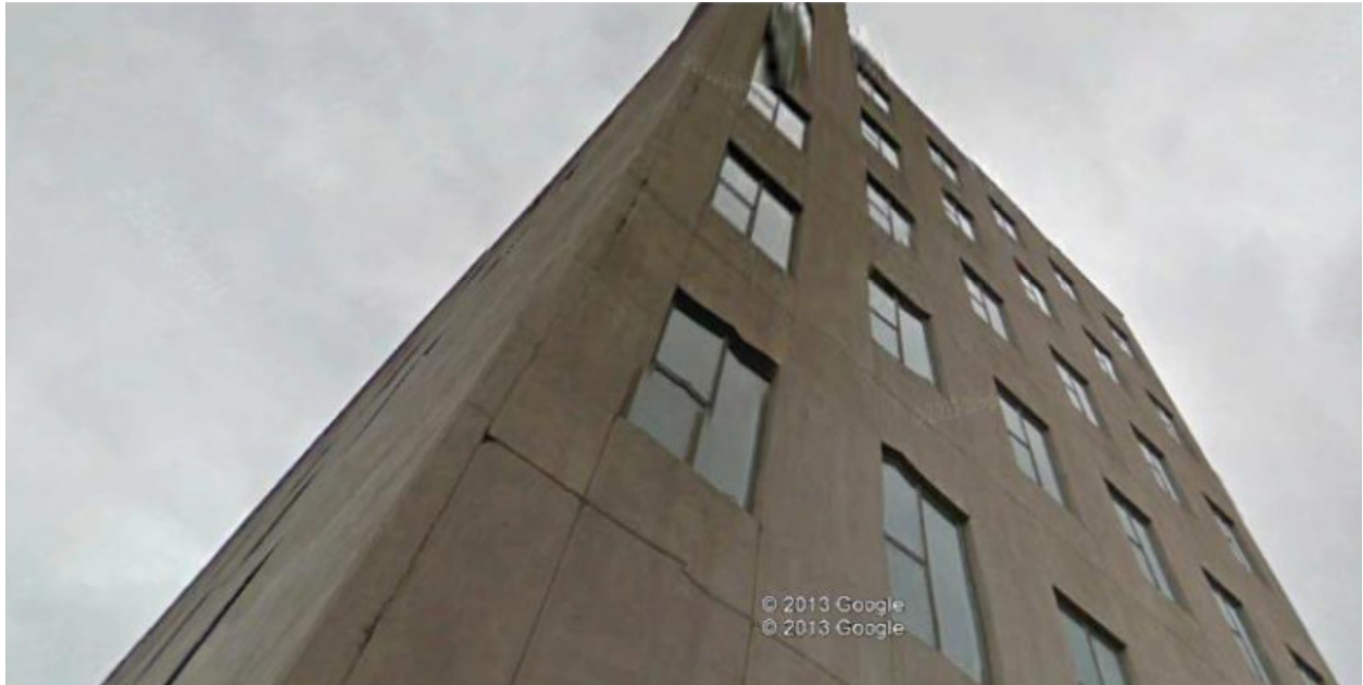
Photo 13: South elevation looking up
