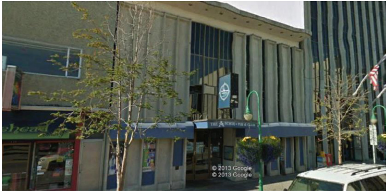
Photo 31: Anchor Pub Entrance
