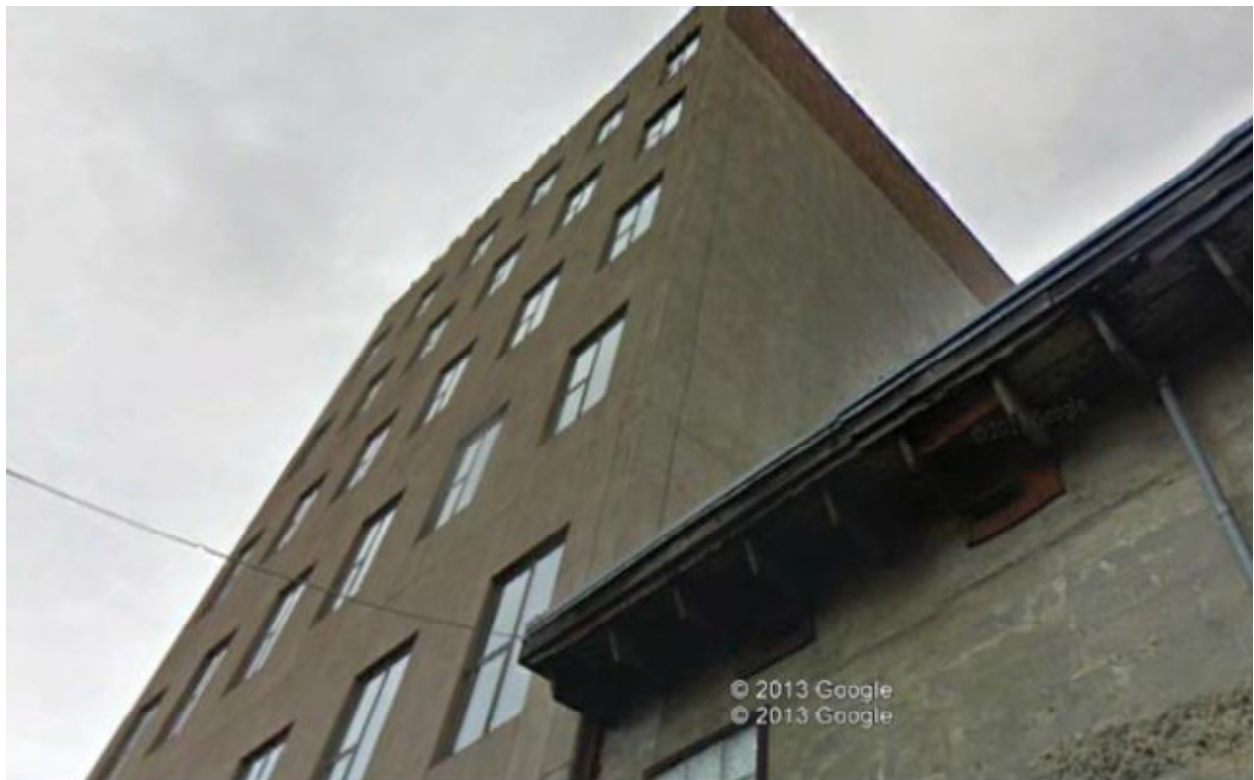
Photo 14: Southwest corner looking up
