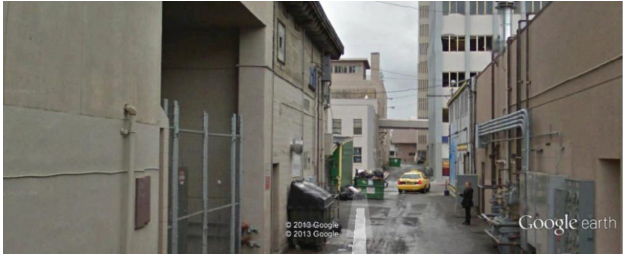
Photo 28: Utilities in Alley behind LIO
