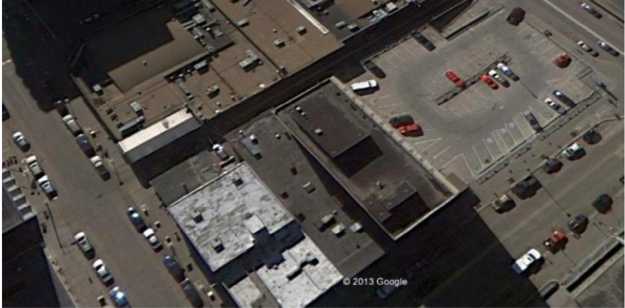
Photo 3: Ariel view #3 Roof and Parking Lot
