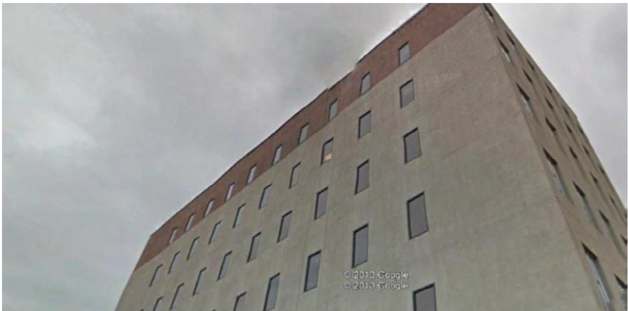
Photo 12: Southwest Corner looking up
