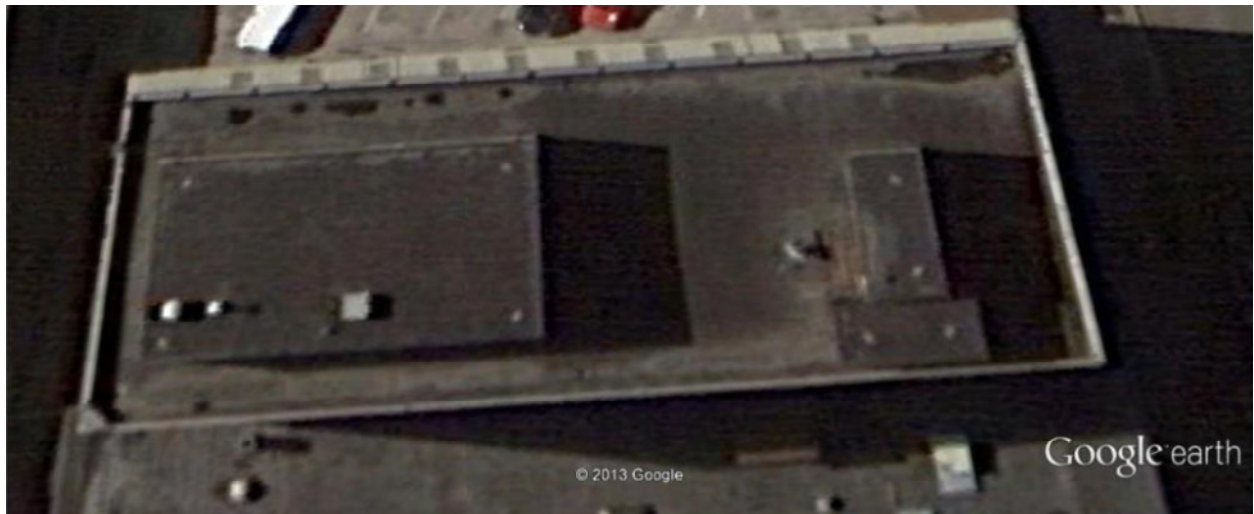
Photo 5: Ariel View #5 LIO Roof
