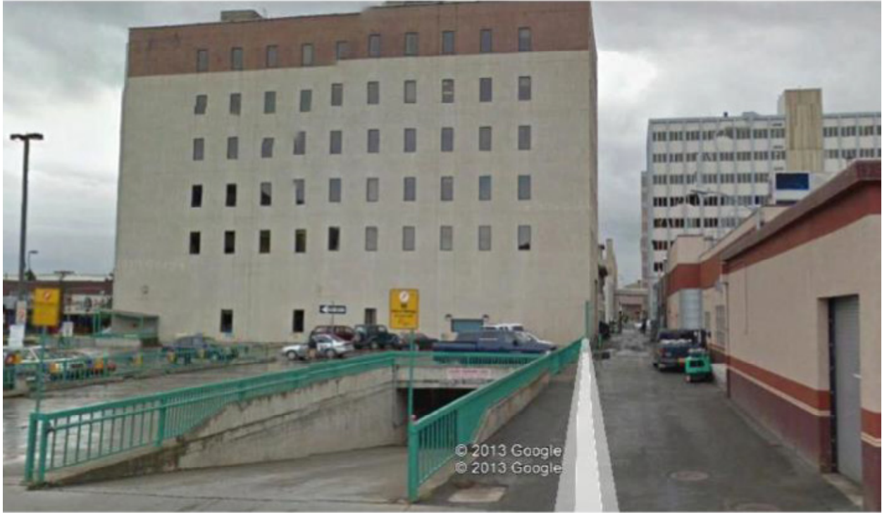
Photo 20: Parking Ramp and Alley
