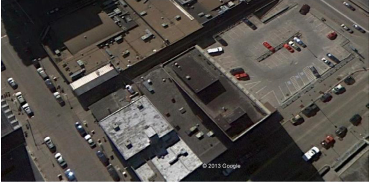
Photo 3: Ariel view #3 Roof and Parking Lot
