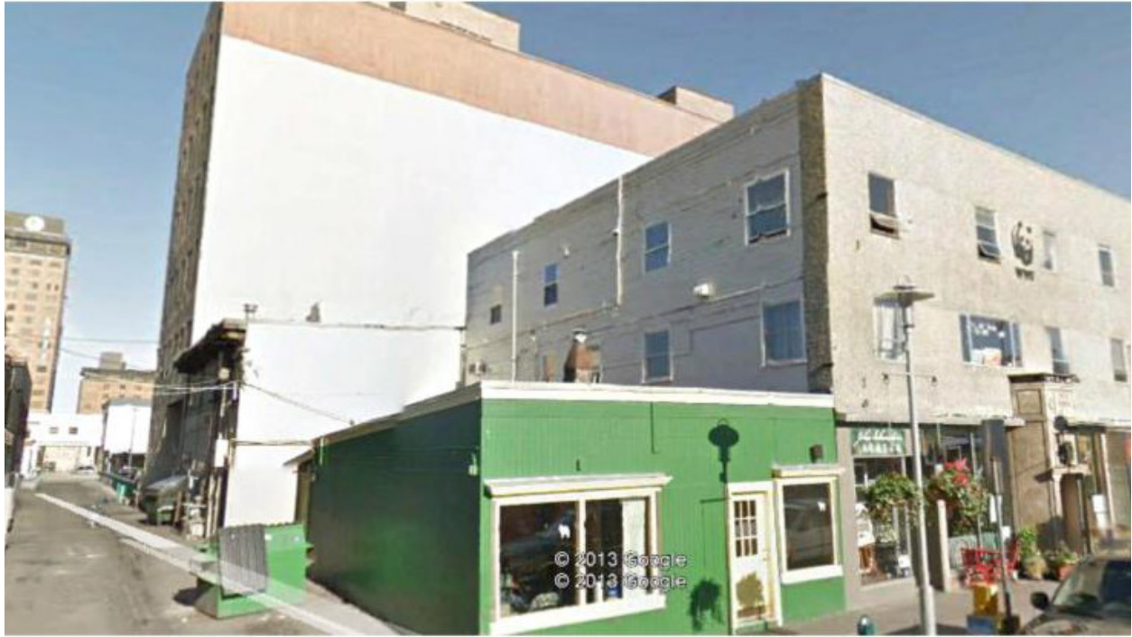
Photo 22: West elevation from G street
