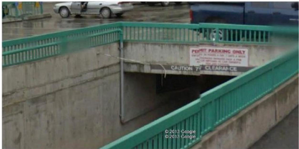
Photo 21: Parking Garage Close up
