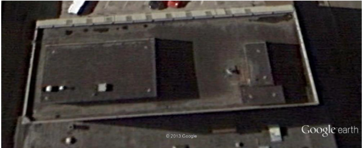
Photo 5: Ariel View #5 LIO Roof
