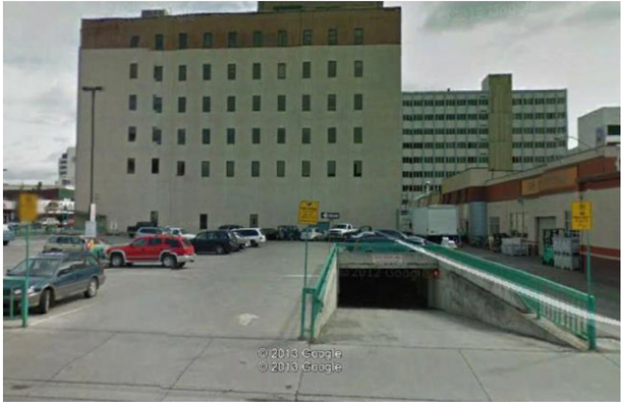
Photo 18: Parking Ramp and West Elevation
