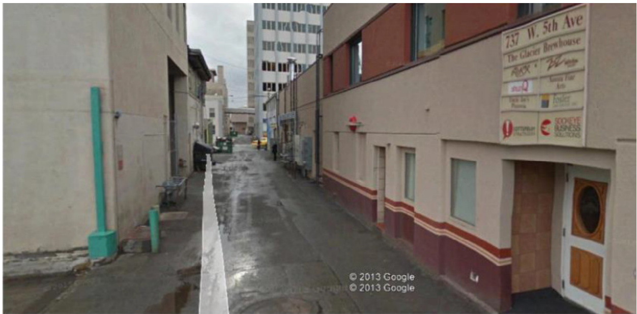
Photo 27: Alley view behind LIO
