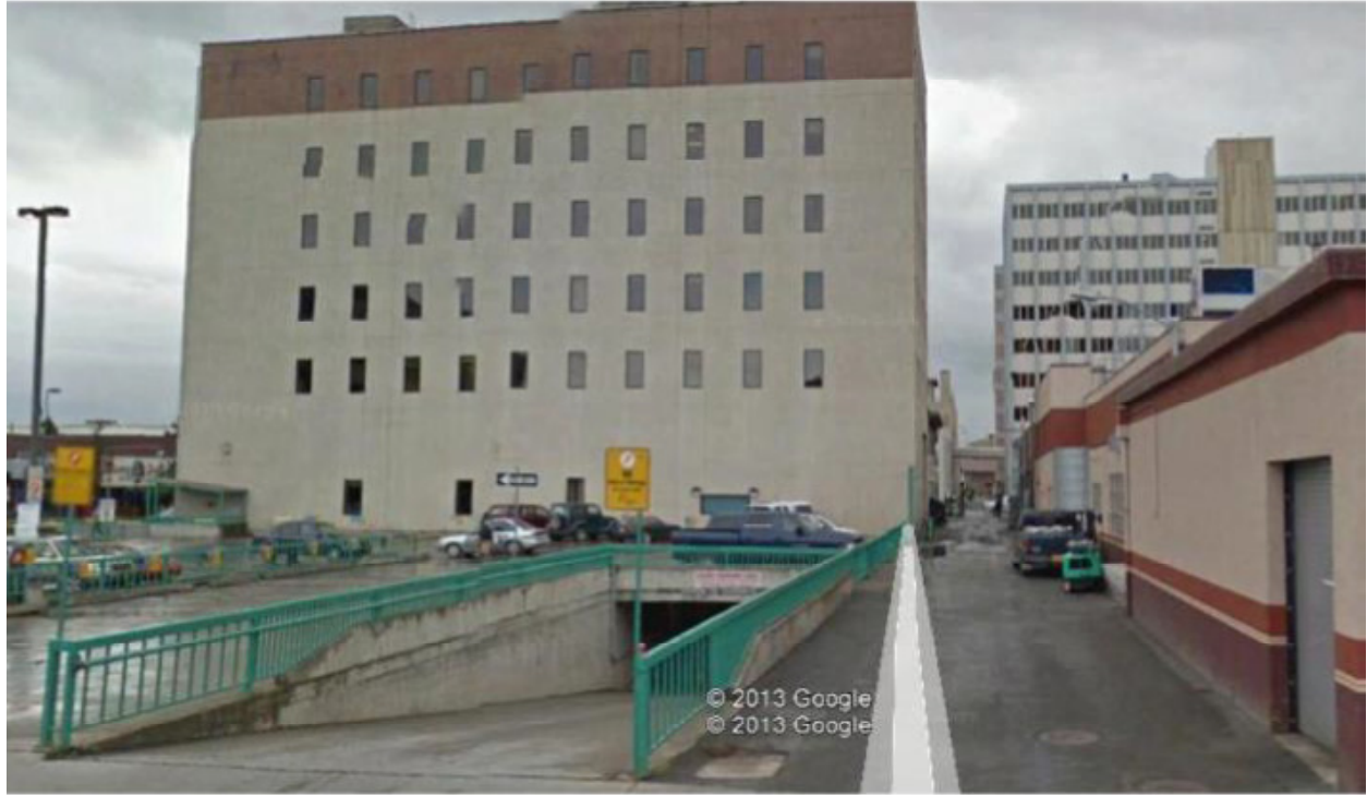
Photo 20: Parking Ramp and Alley
