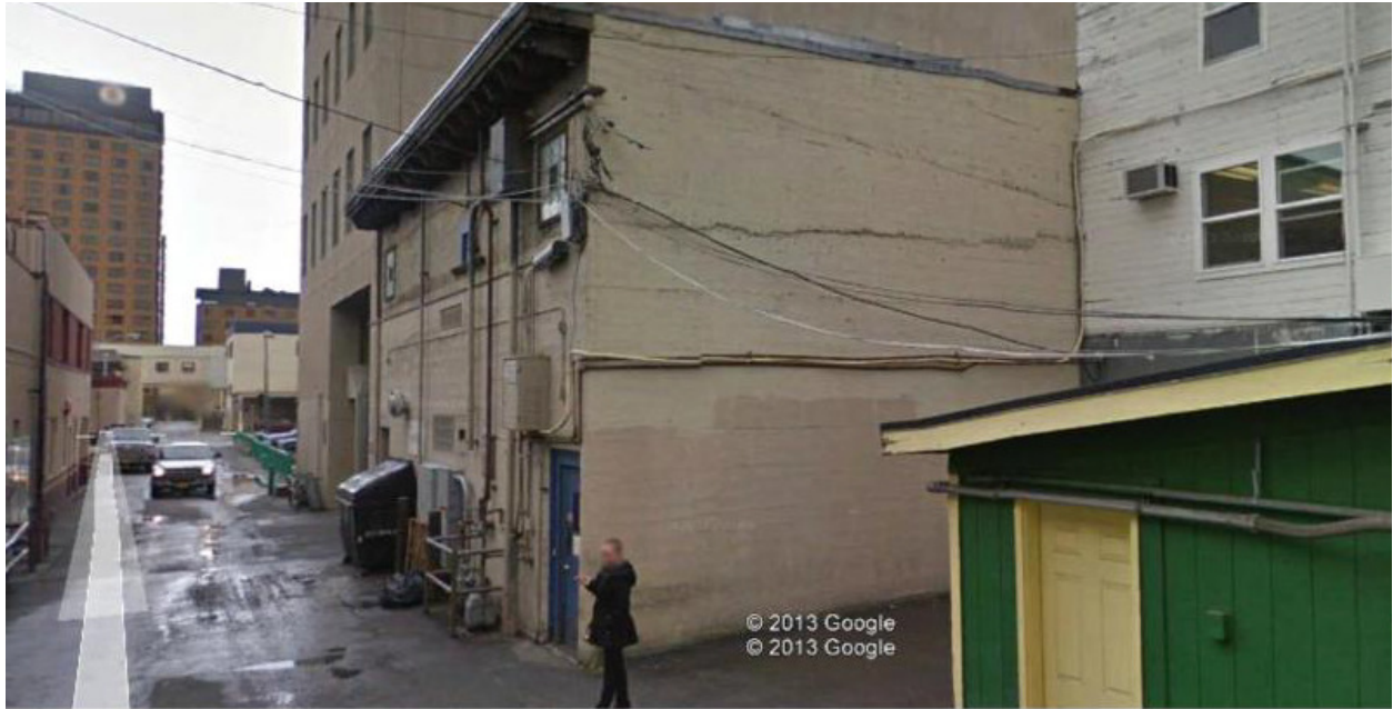
Photo 30: South End of Anchor Pub Building
