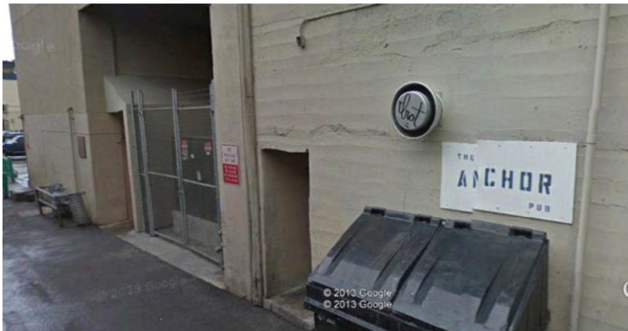
Photo 29: South Wall of Anchor Pub
