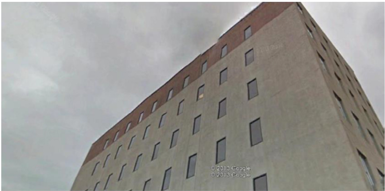
Photo 12: Southwest Corner looking up
