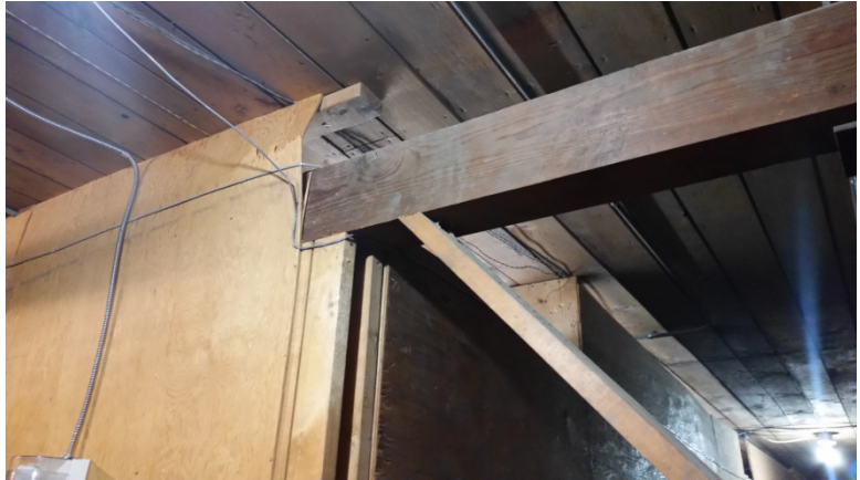
Figure 5 Buckled plywood
