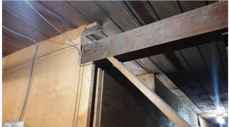
Figure 5 Buckled plywood
