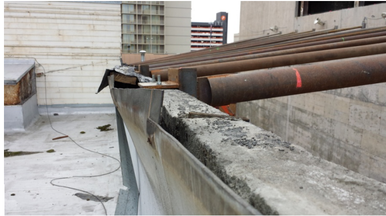
Figure 12 Open top of common wall
